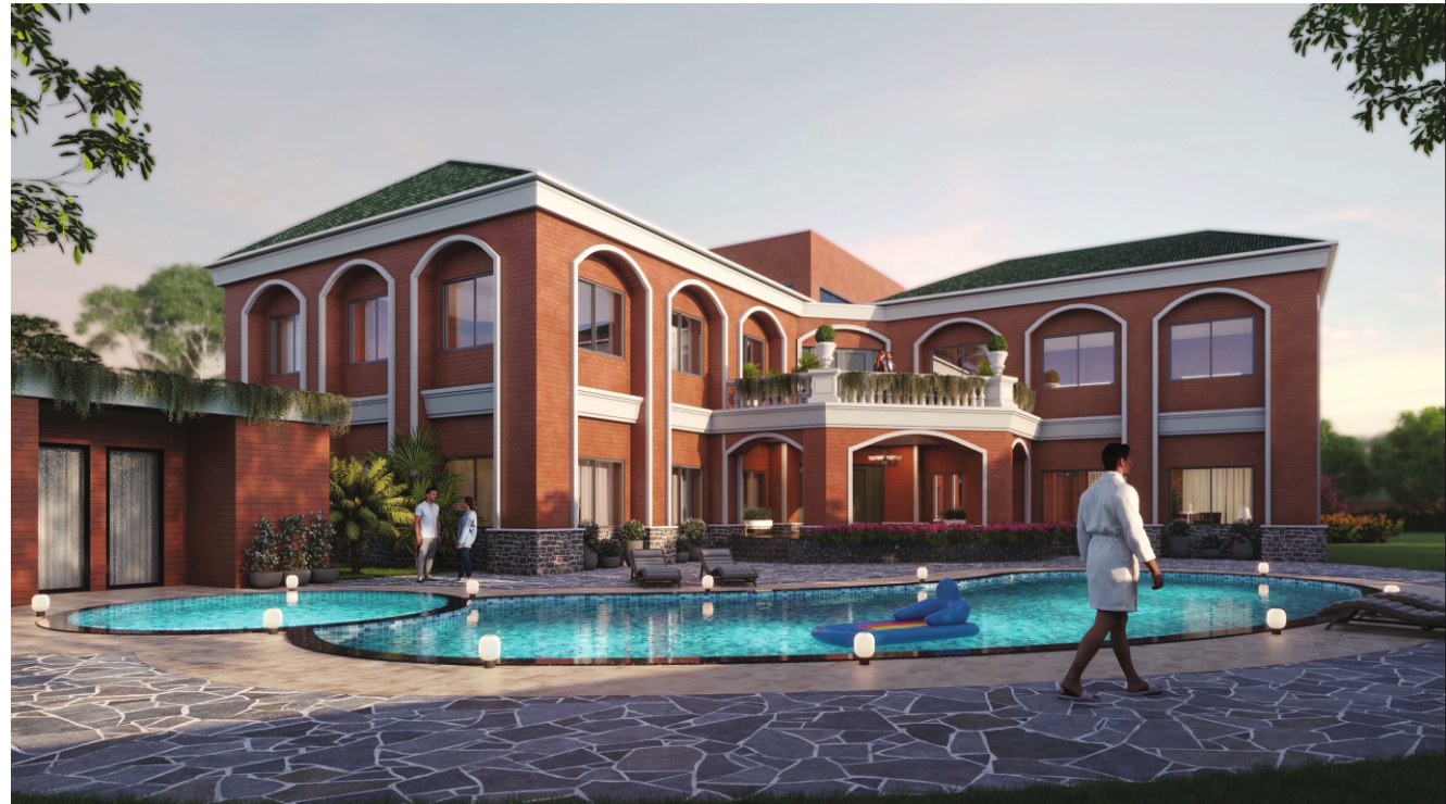
Club House with pool view at The Future City
